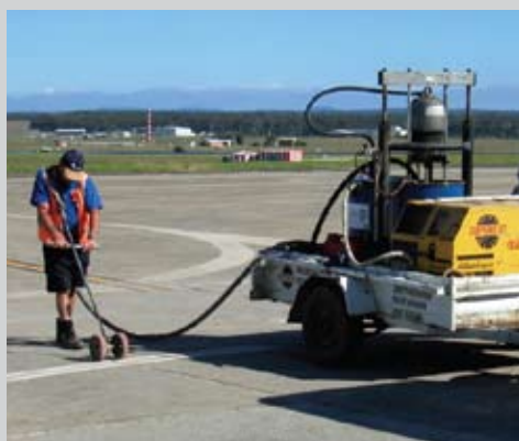
Joint resealing at HMAS Albatross
