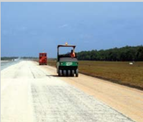
Rolling a bitumen emulsion sand seal, Lockhart River Airport
