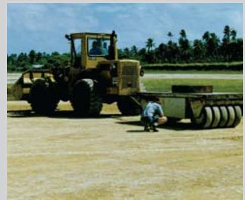
Proof rolling pavement in Ha'apai, Tonga
