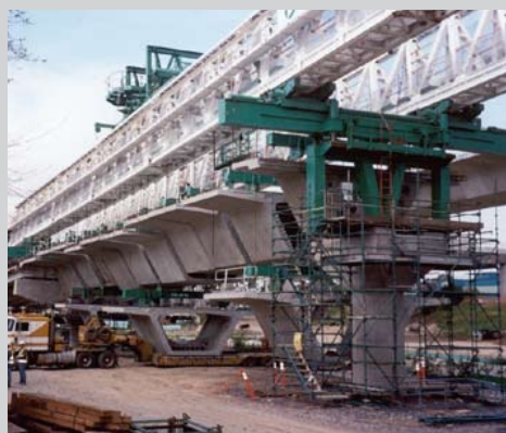
Ramp erection using overhead gantries, Western Link Viaduct
