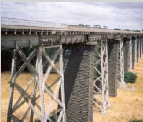
Moorabool rail viaduct, assessed for long-term maintenance requirements
