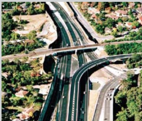
M2 Motorway, linking Sydney's inner city with the north-west suburbs
