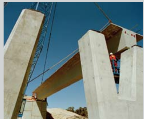
Construction of Welshpool Road Bridge Roe Highway, Sections 4 & 5, Perth
