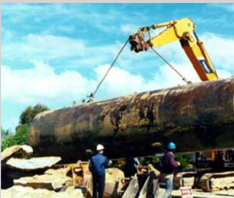
Remediation of fuel facilities.
