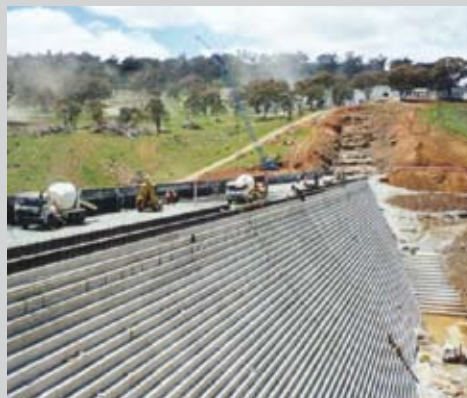
Candangullong Dam, NSW Australia. RCC design and construction advice
