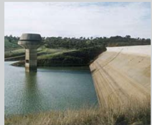
Little Para Dam, SA Australia. Dam safety investigations & remedial works.
