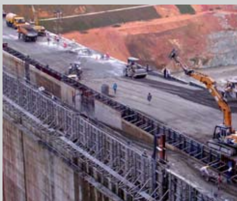
Kinta Dam, Malaysia. Feasibility study, engineering design and project management services.
