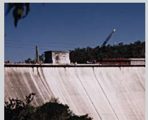
Canning Dam, WA Australia. Dam post tensioning project
