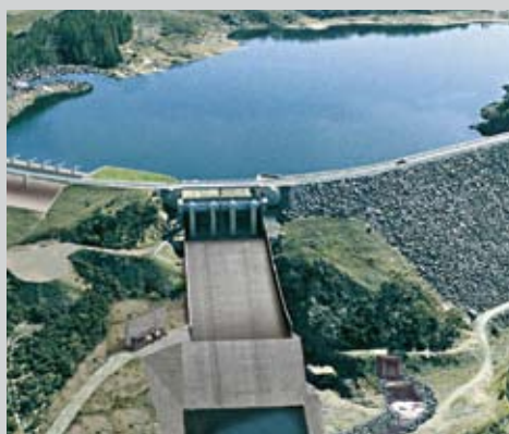
Jindabyne Dam, NSW Australia. Auxiliary spillway
