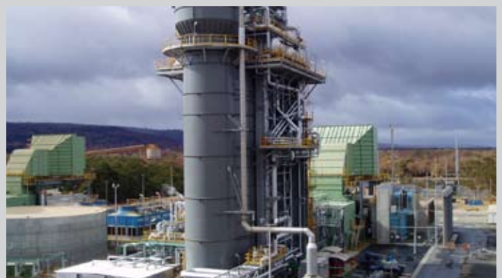
Alinta's 2 x 140MW cogeneration at Alcoa's Pinjarra refinery, Western Australia
