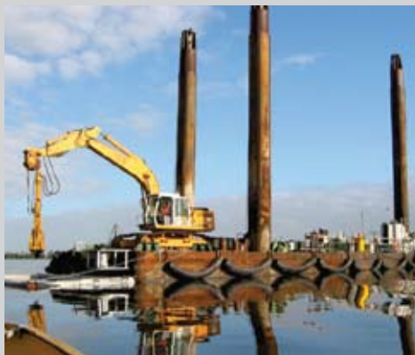
Dredging of the South Arm of the Hunter River, NSW, Australia.
