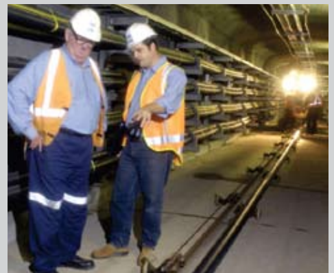
Electricity Supply Augmentation Project, Sydney CBD, NSW, Australia.
