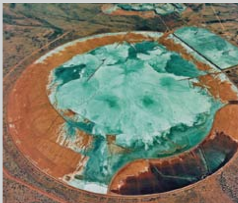
Tailings dam - Mt Keith.
