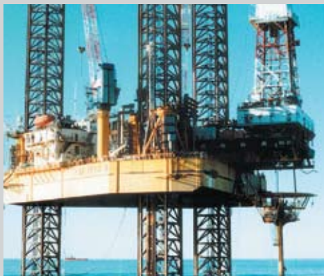
Hakuryu Oil Rig positioning, Barrow Island, WA
