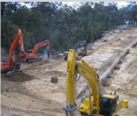
Construction - Mallaty Creek Pipeline, NSW
