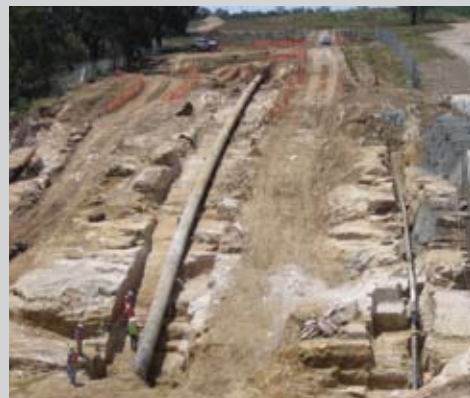
Pipe relocation - Mallaty Creek Pipeline, NSW
