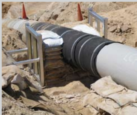
Temporary pipe support- Mallaty Creek Pipeline, NSW
