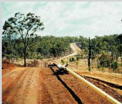
Wide Bay Pipeline, QLD
