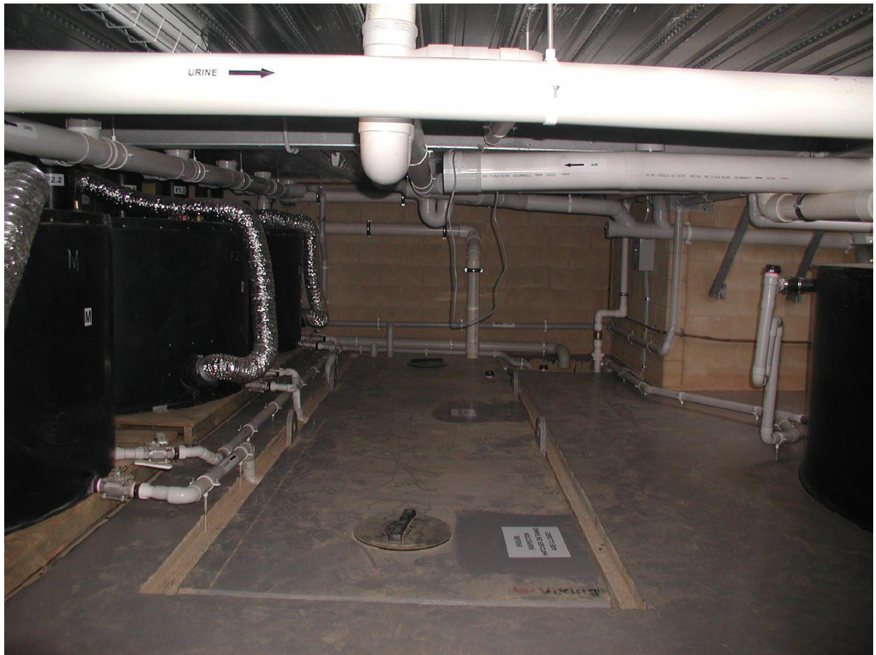
Figure 3 View inside basement
