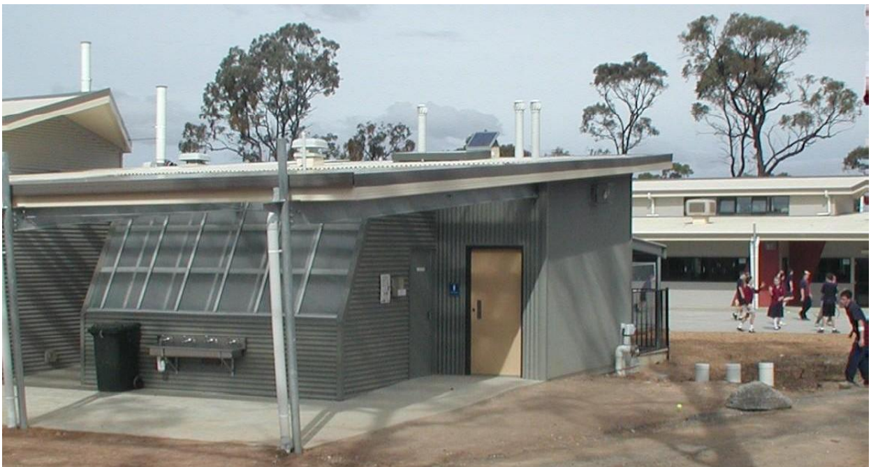
Figure 2 Outside view of structure from the West
