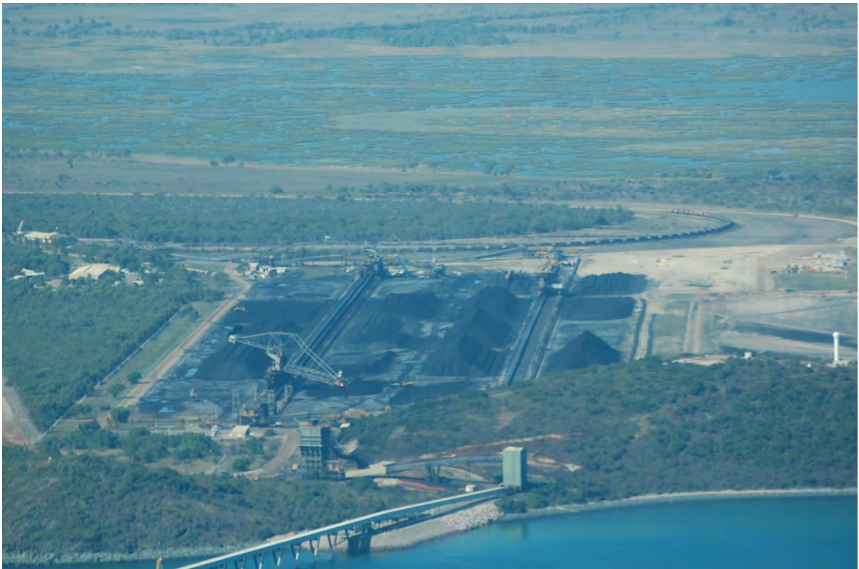
Photo 3-1 Oblique view of existing Abbot Point Coal Terminal
