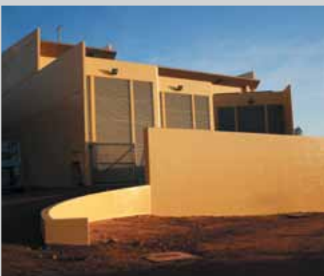
Frances Bay Zone Substation
