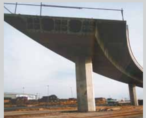
Bagot Road Bridge
