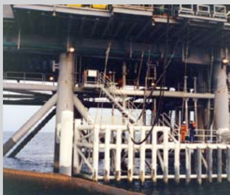
CP audit of platforms, pipelines, mooring, floating production and storage
