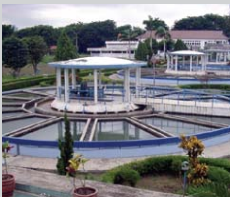
Water structures maintenance investigation, repair and maintenance audits
