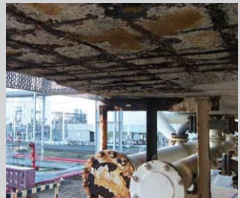
Industrial structures investigation and repair
