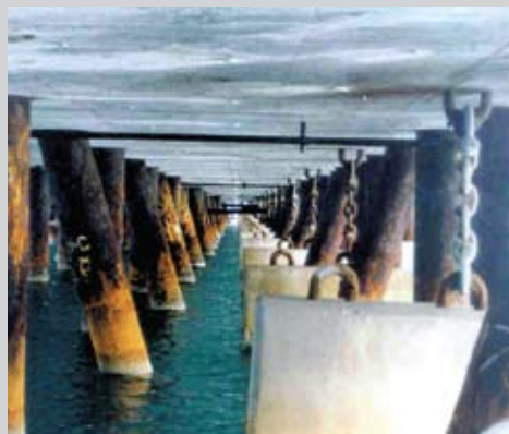
Marine structures investigation, repair (including CP), corrosion monitoring and maintenance audits
