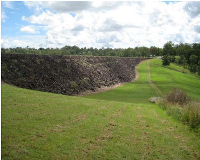
**Figure 1. Maroon Dam downstream berm and embankment**
