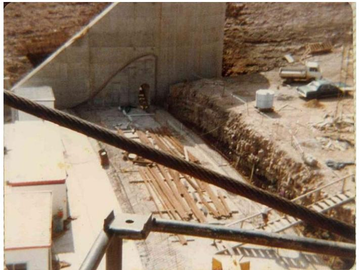
Figure 10 Original ogee construction, showing rock excavation
