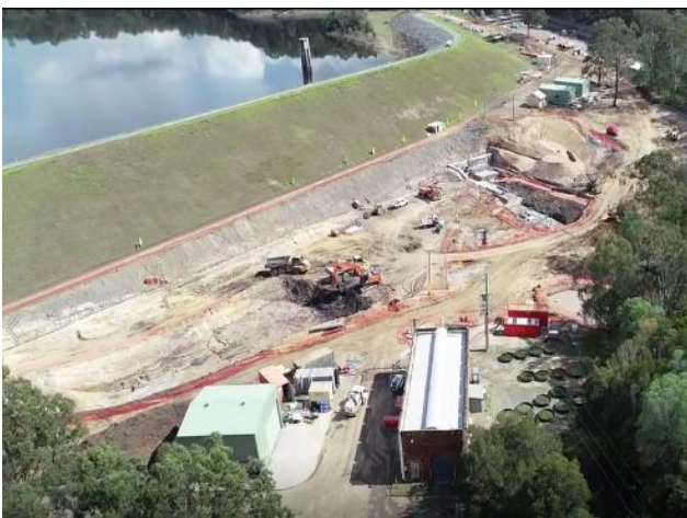
Figure 4 - Excavation at toe (looking upstream)
