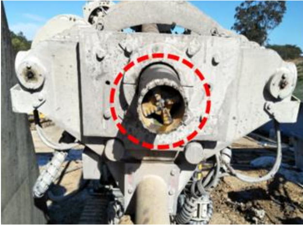
Figure 2 - Drill head showing casing (circled) and wash bore bit
