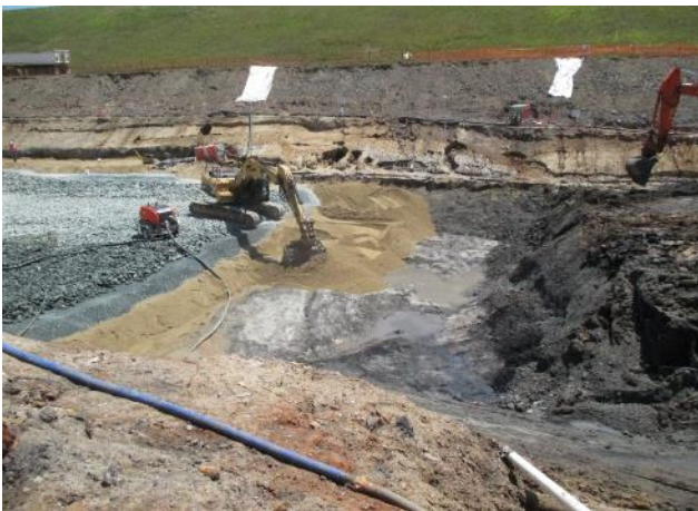
Figure 8 - Simultaneous excavation and backfill
