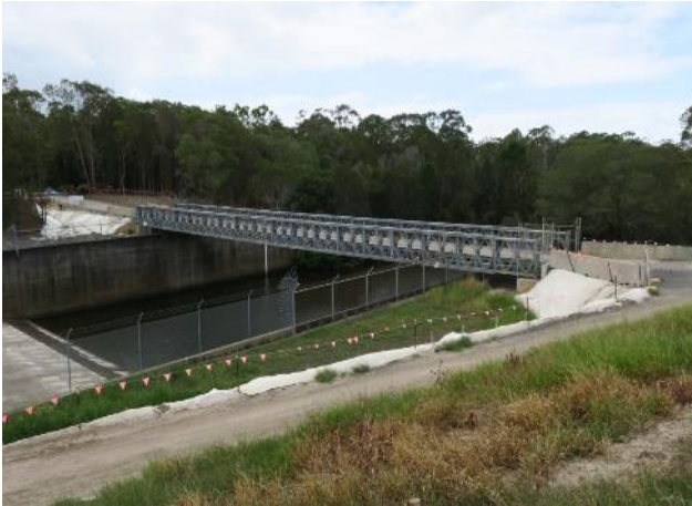
Figure 9 - Temporary access bridge over spillway
