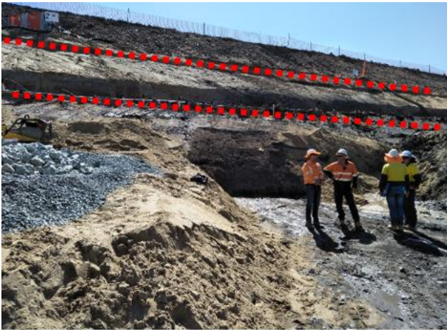
Figure 6 - Double row of dewatering wellpoints (indicated as shown)
