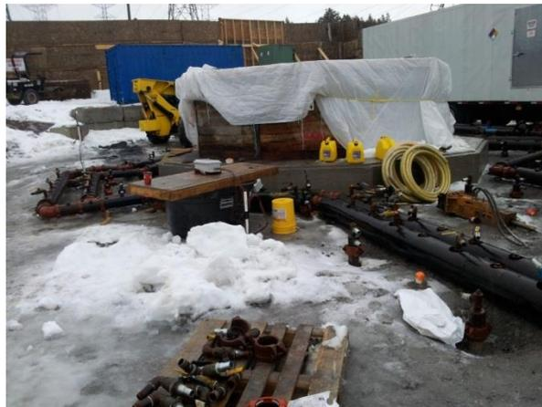
**Figure 7 Southeast Collector Shaft 11 Ground Freezing Setup**
