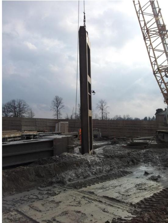
**Figure 5 Diaphragm Wall Construction on the Southeast Collector**
