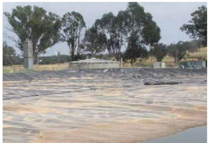
**Figure 2. A covered anaerobic lagoon can potentially be used to generate electricity from gas while providing treatment during vintage.**
