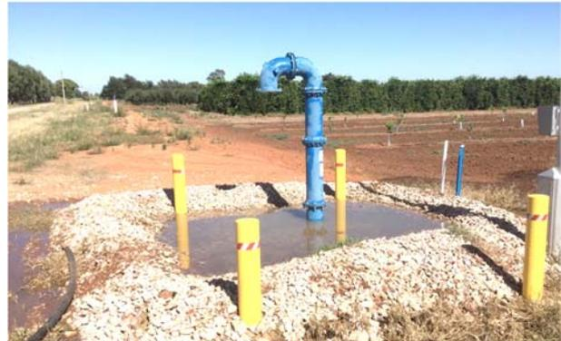
*Figure 4: Standpipe at a surge-prone location with flooded surrounds, prior to flow-control modifications.*
