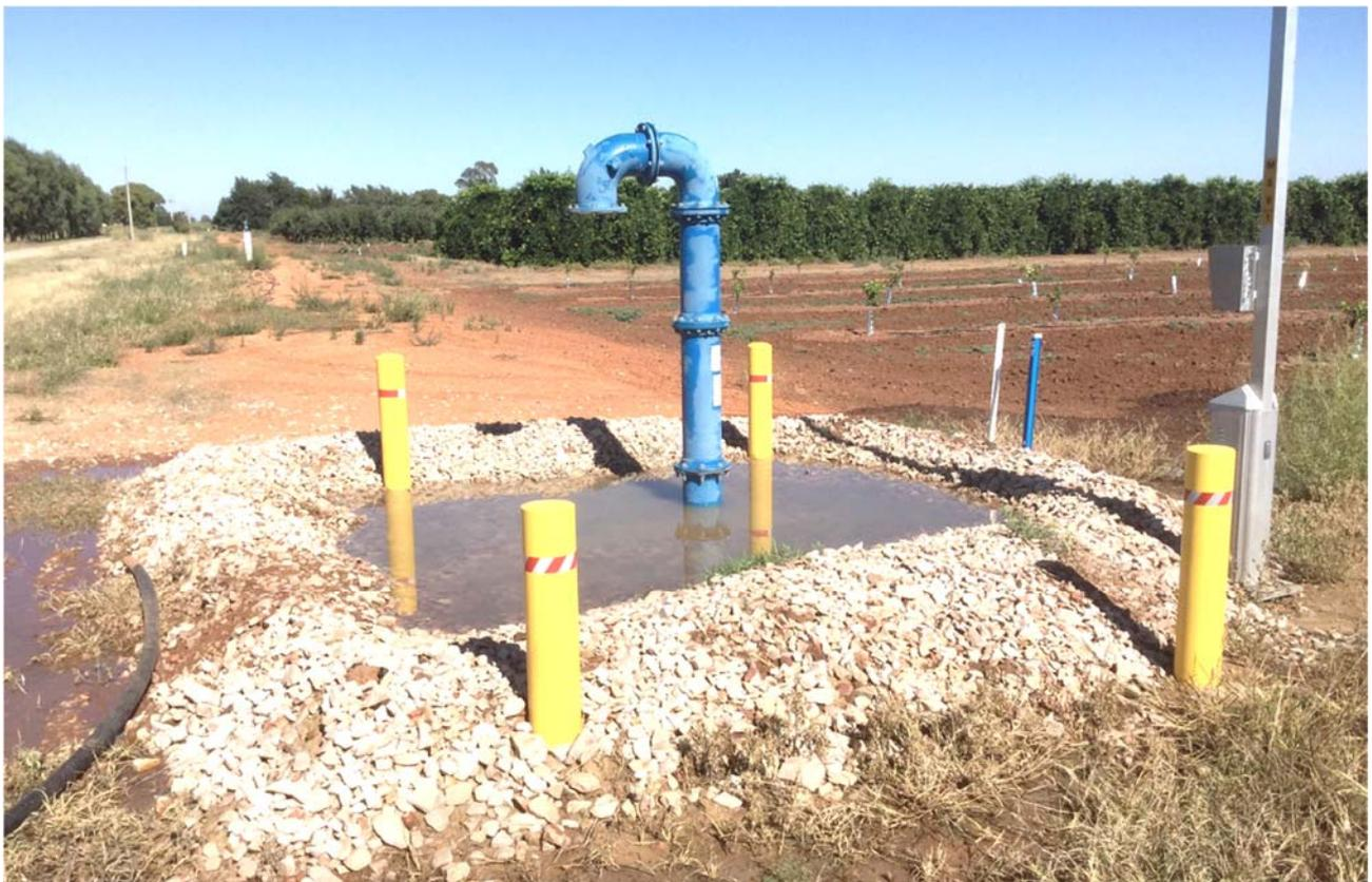
Figure 1: Standpipe installed at a surge-prone location
