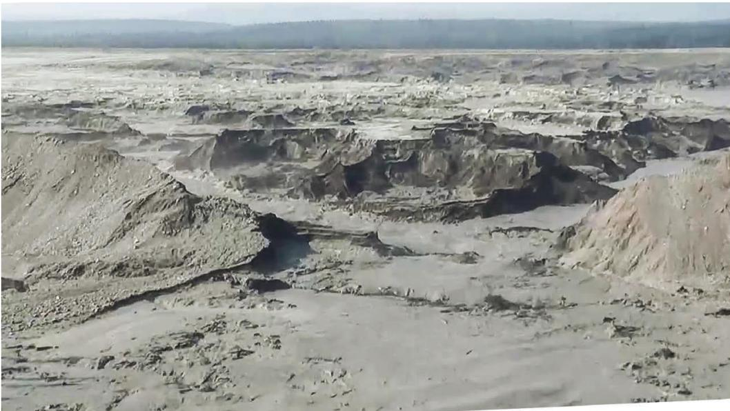
**Figure 1** View of the Mt Polley Tailings Dam Failure
